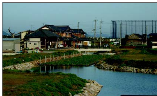
Fig. 10.2 Constructed wetland for surface runoff from arable land, Japan (photo: V. Santiago-Fandino)
