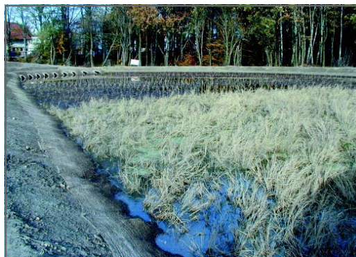
Fig. 10.1 Constructed wetland for storm water Karls-Einbau Project Company (photo: EKON Polska Biologia Inzynieryjna Sp. z o.o.)
